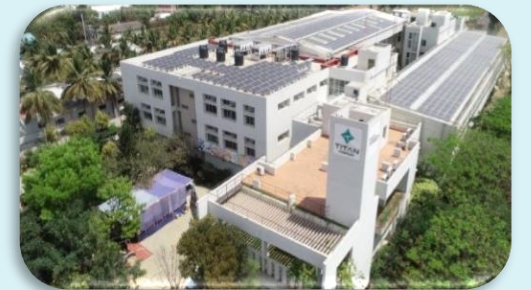
Manufacturing facility at Chikkaballapur
