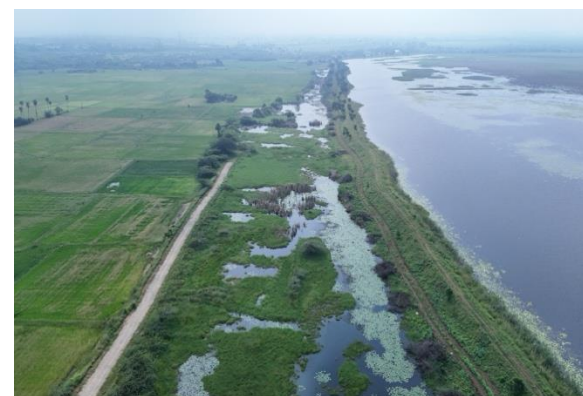
Kanchipuram Lake Rejuvenation work
